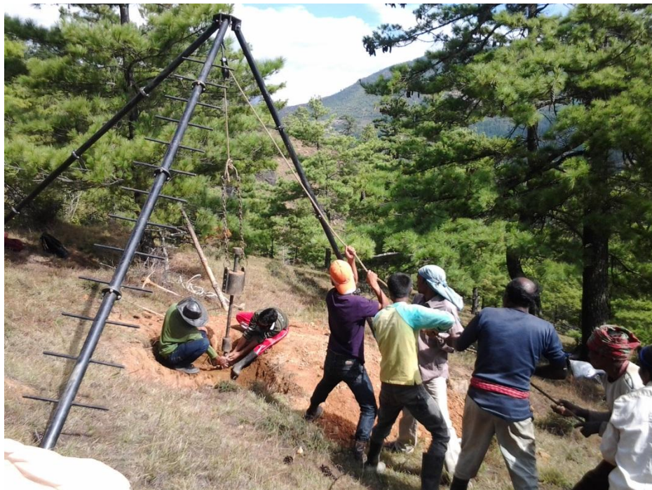
Fig. Standard Penetration Test set up
