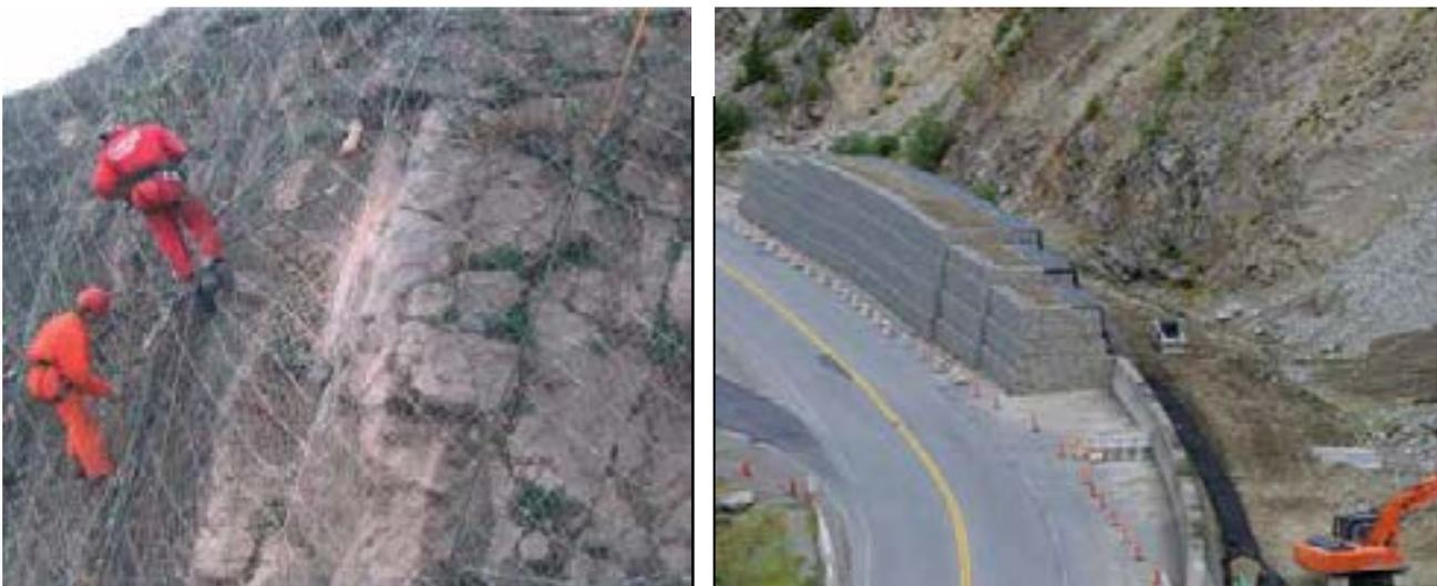
*Implementation of suitable countermeasure works for rock slope failure (Rockfall)*
